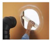
3- You must first secure the wall thimble into the exterior wall surface. Then, do the same inside and fasten the trim plate.
